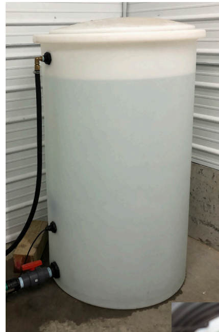
250-gallon holding tank, with brass float valve and supply plumbing
